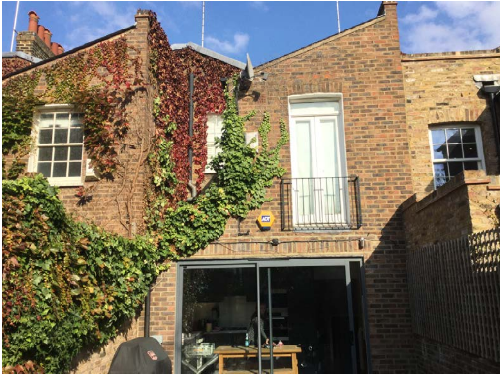
Rear elevation of 62 Bourne Street
